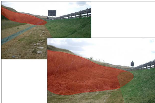
Figure 42. A16: km 112+400 site
