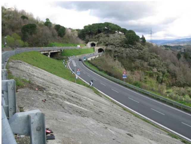
Figure 40. Piano d'Infante site: concrete panels between roadways to be equipped with SMAMID and POIS system
