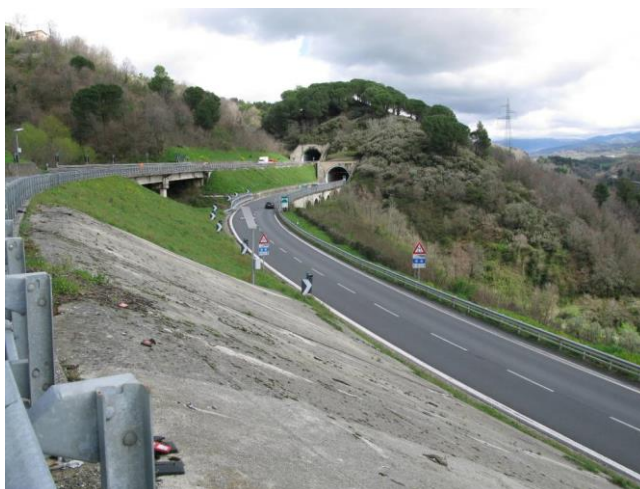
Figure 39. Piano d'Infante site: concrete panels between roadways to be equipped with SMAMID and POIS system
