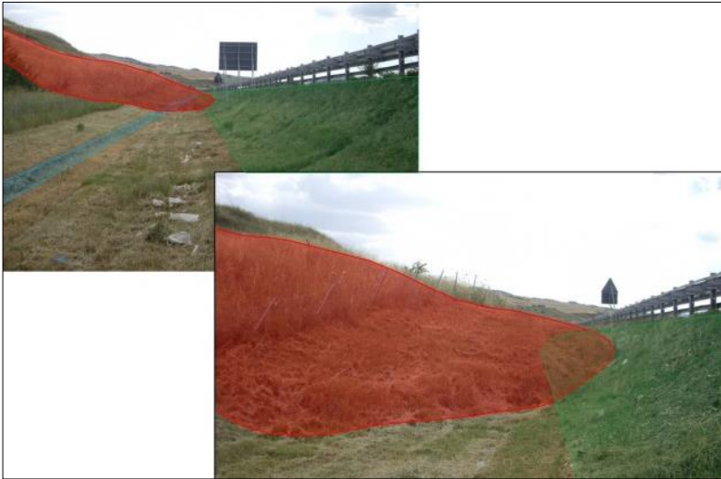
Figure 41. A16: km 112+400 site
