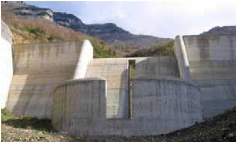
**Figure 24. Upstream open check dam in the Cantariello gully in Sarno**
