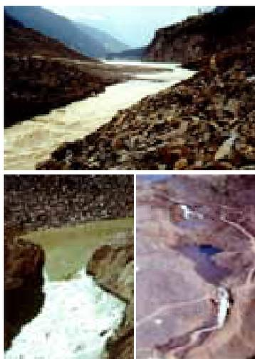
Figure 18. Artificially controlled overflow of the Val Pola lake
