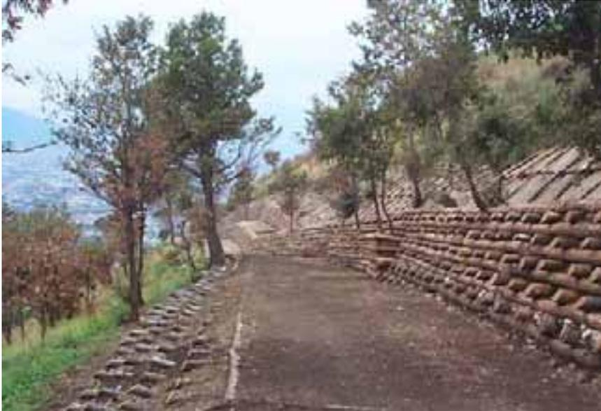
**Figure 19. Example of bioengineering works along Pizzo d'Alvano side**
